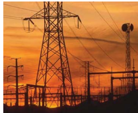
Transmission & distribution loss
